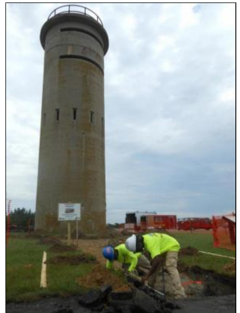
Kent Construction's Ron Summers and Mike Derrickson run a string before work can begin on a new sidewalk. CHRIS FLOOD PHOTO
